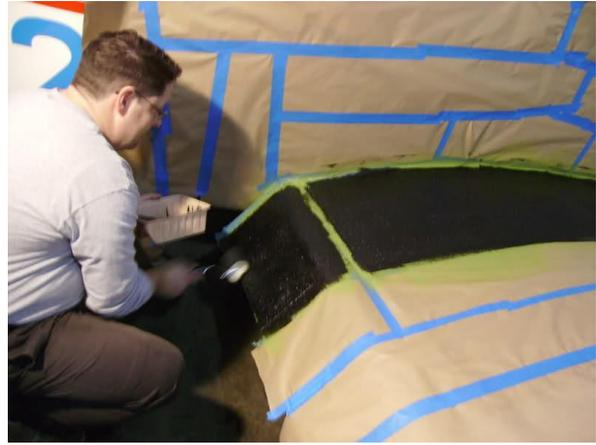
Once applied with a brush, I went back over the UltraWing Walk with a roller to ensure even distribution and no brush marks.
